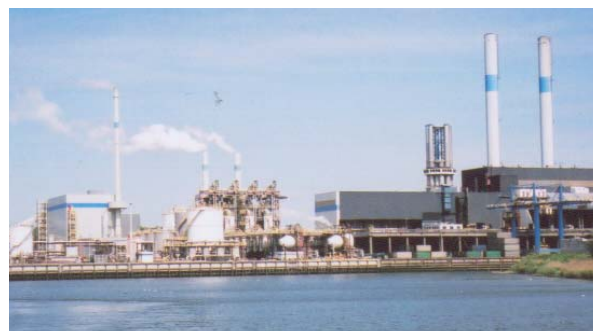
The AVR Waste-to-Energy plant at Rozenburg is one of the biggest waste incineration plants in Europe. On the same site, the new biomass energy plant (left) converts 150,000 t/a of demolition wood into 192 GWh/a of green electricity. Courtesy Mr Andre Rekveld, the Netherlands.
