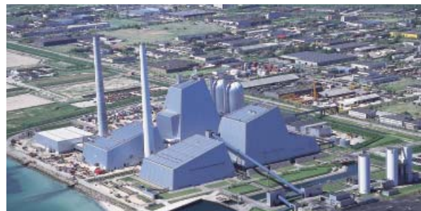
Avedøre Power Station, a 570 MW multi-fuel plant that can utilise natural gas, oil, and biomass in the form of straw, wood pellets and wood chips. Courtesy Thomas Scott Lund, Energi E2, Denmark.
