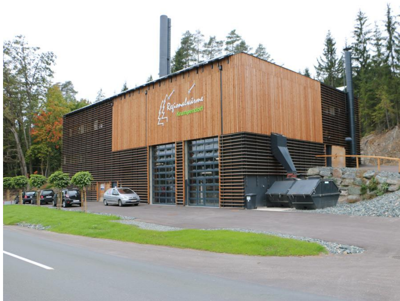
Biomass heating plant Krumpendorf, Austria
