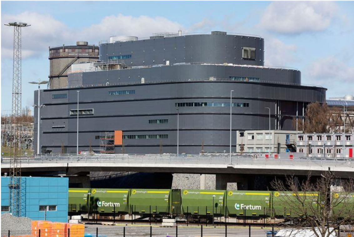
Värtaverket biofuelled CHP plant in Stockholm
