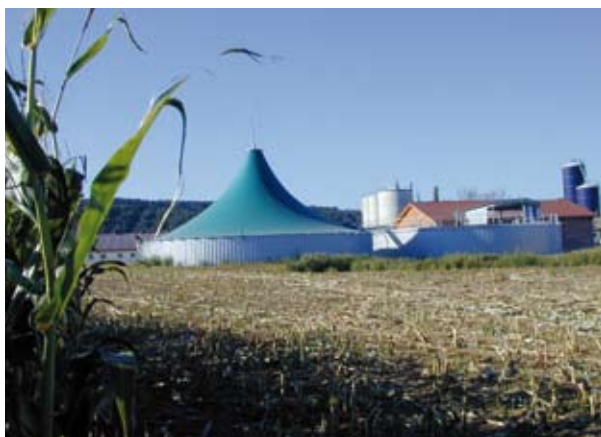
Photo 11: General view of a 2-step crop digestion plant with digester 1 (right) and combined gas collector and digester 2 (left)
