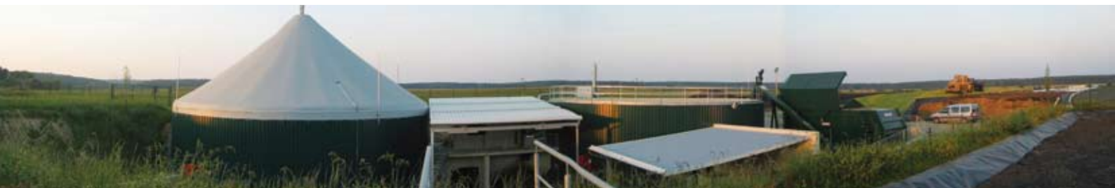
Photo 13: General view of a two-step, 500 kW e only energy crop digestion plant with digester 1 and dosing unit (center), digester 2 with integrated gas holder (left), silage clamps (background) and storage lagoon for the digestate (foreground right).
