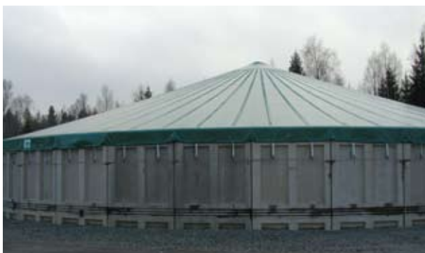
Photo 9: Gas tight coverage of a post storage tank for digestate in Sweden. Residual biogas developed from digestate is collected for energy use, while greenhouse gas and ammonia emissions are prevented.
