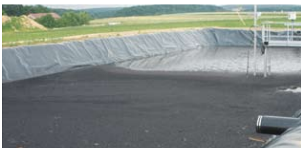
Photo 10: Open lagoon storage for completely digested maize and grass silage; this is applicable where there is no longer any possibility for methane production from the digestate
