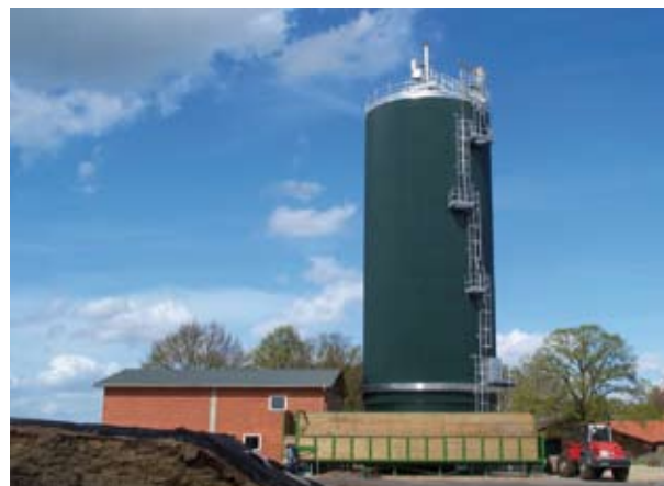
Photo 15: Dry continuous digestion
