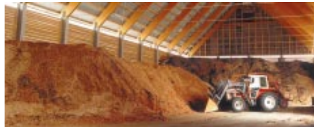
Wood chips storage facility for biomass district heating plant, Bad Mitterndorf/Austria. (Courtesy of LEV, Austria)
