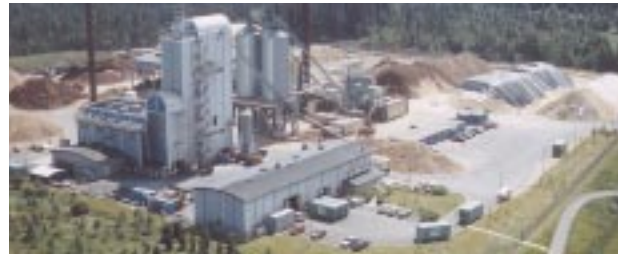
The IGCC plant in Värnamo/Sweden is the first thermal biomass gasification plant worldwide, with a substantially increased power-to-heat ratio relative to conventional boiler/steam turbines. (Courtesy of Sydkraft, Sweden)
