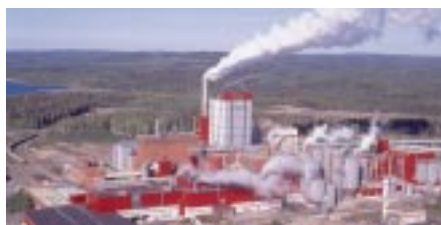
The Enocell Pulp Mill, Uimaharju/Finland, is a modern chemical pulp mill which produces excess heat and power by using process wastes as fuel. (Courtesy of Enso Group, Finland)
