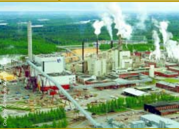
Alholmens Kraft CHP plant, Pietarsaari, Finland. The largest biofuelled power plant in the world.
