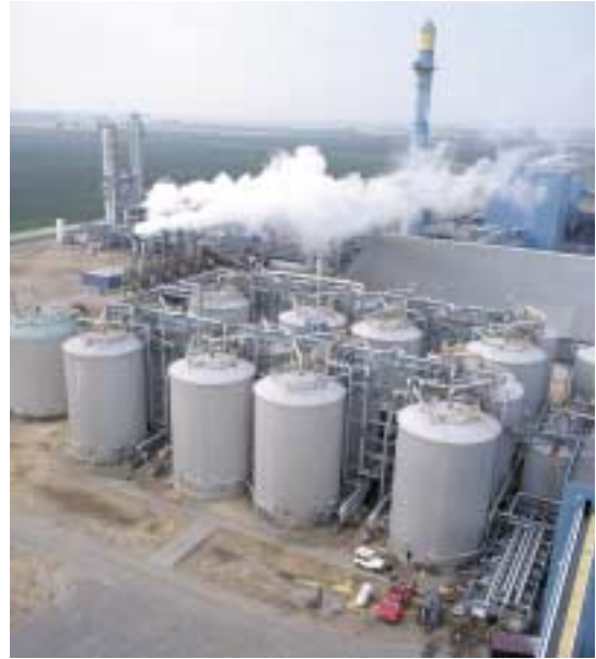
Ethanol pilot plant based on corn fibre and other cellulosic material, New Energy Company of Indiana, USA. (Courtesy DOE/NREL and W. Gretz)
