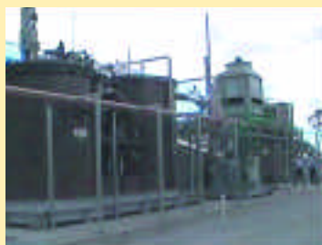
Greenwaste gasifier, currently being installed at Whytes Gully Landfill, Wollongong, NSW.
