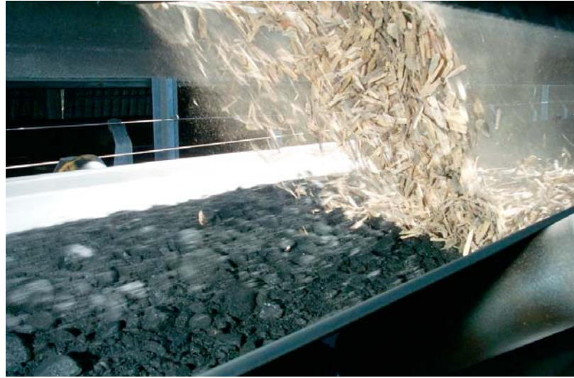
Dumping wood chips on a coal conveyer before the mills. Courtesy Delta Electricity, Australia.
