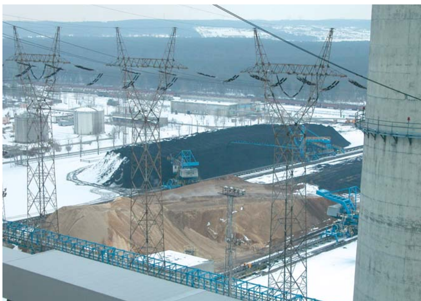
Biomass and coal fuel storage facilities at the Dolna Odra co-firing plant in Poland. Courtesy I. Obernberger, Bios-Bioenergy, Austria
