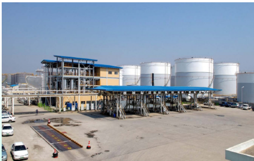
Overview of Biodiesel Plant
