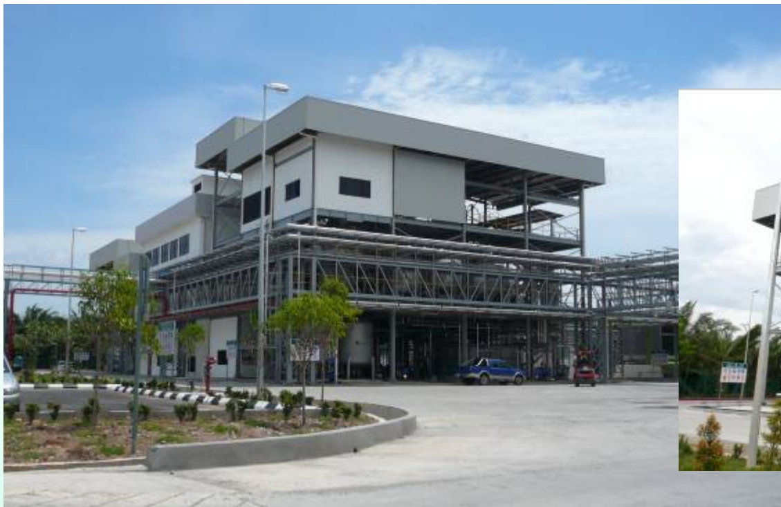
Normal-grade Palm Biodiesel Plant 60,000 TPA
