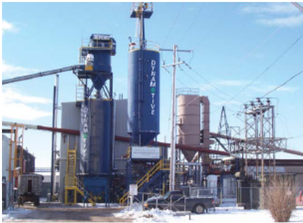
Dynamotive 100 t/d fluid bed fast pyrolysis plant, Canada
