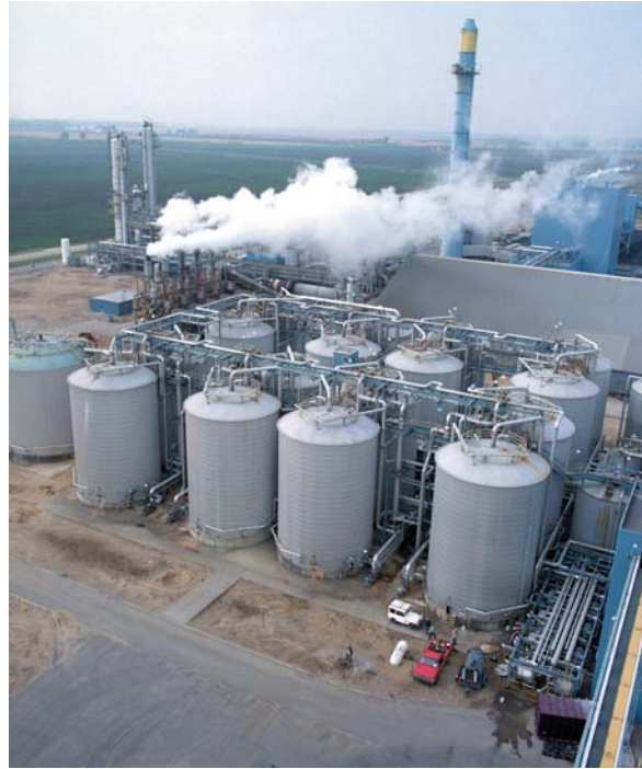
Ethanol pilot plant based on corn fibre and other cellulosic material, New Energy Company of Indiana, USA. (Courtesy DOE/NREL and W. Gretz)
