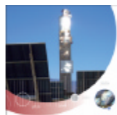
Concentrated Solar Power
