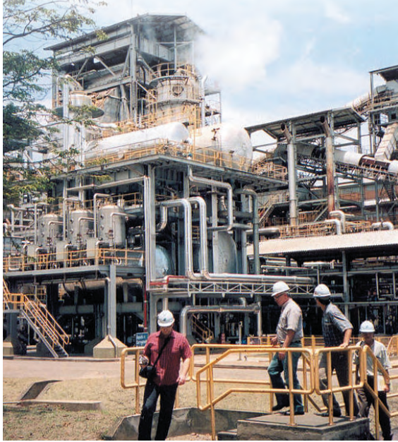
The Barra Grande alcohol and sugar production plant in Brazil produces ethanol from sugar cane on a commercial scale
