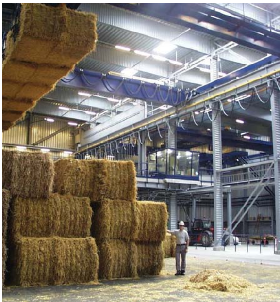
Denmark – Avedøre 2's straw boiler burns 1200 bales per day. Courtesy Thomas Scott Lund, Energi E2, Denmark.
