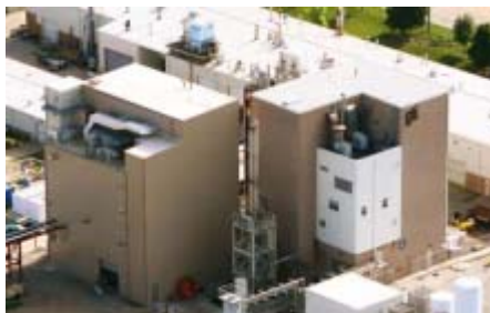
Pilot Scale Gasification Campus
