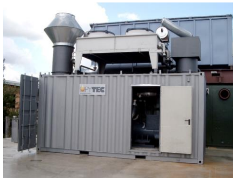
Pytec has tested Bio-oil in a modified 450 kWe diesel engine
