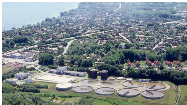
Figure 1: General view of Fredericia WWT-plant. Source: Fredericia Rensningsanlæg.
