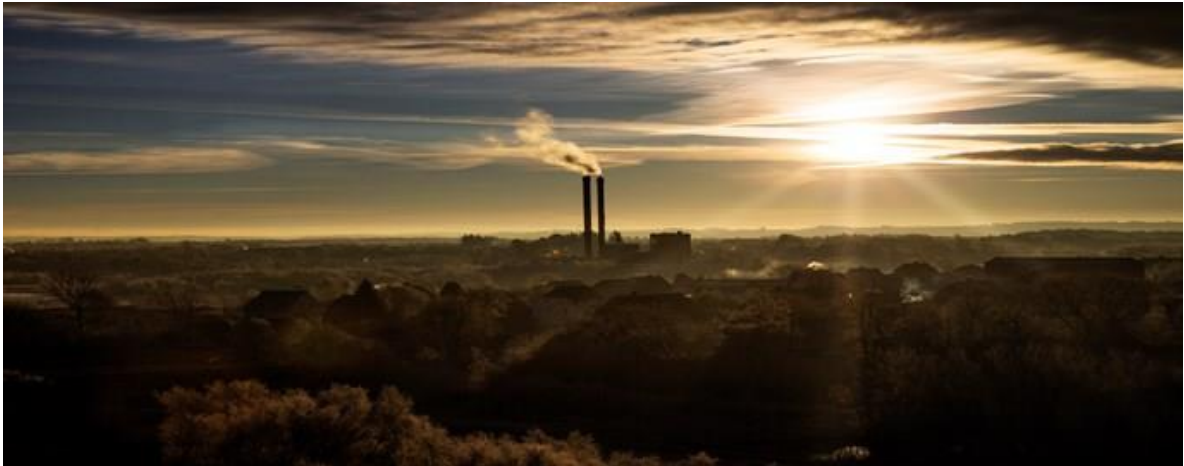
Gasification plant in Skive, Denmark (courtesy of Skive Fjernvarme)
