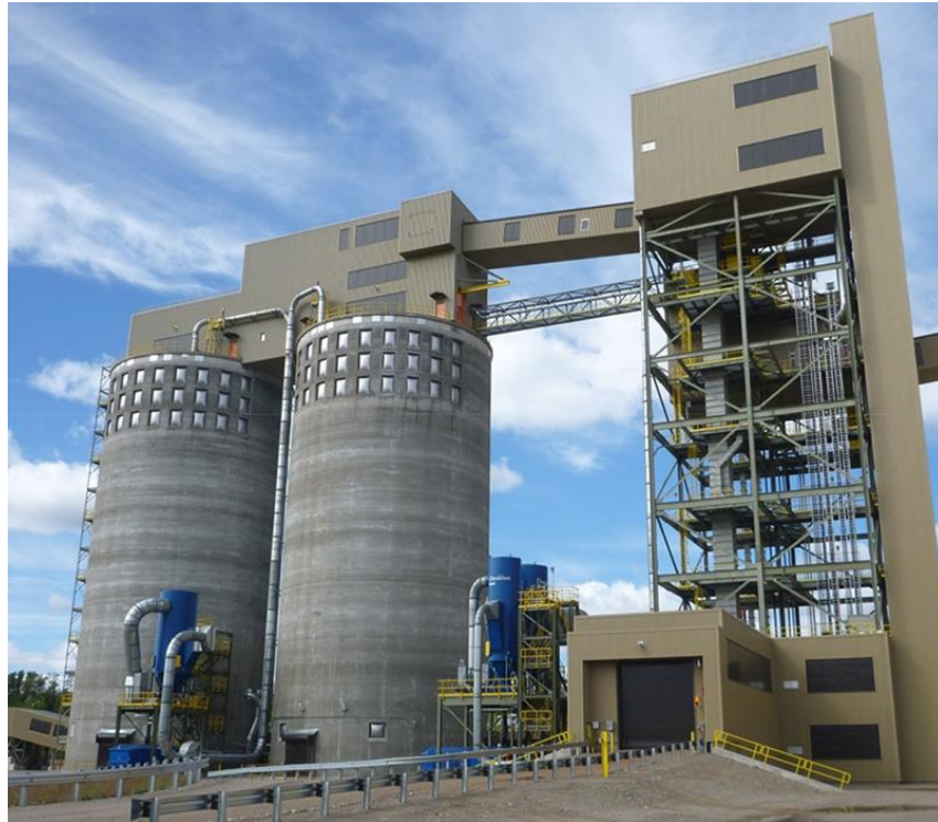
Two new silos were constructed at Atikokan during the conversion to biomass. Each is 44 meters tall, and holds approximately 5,000 tonnes of wood pellets.
