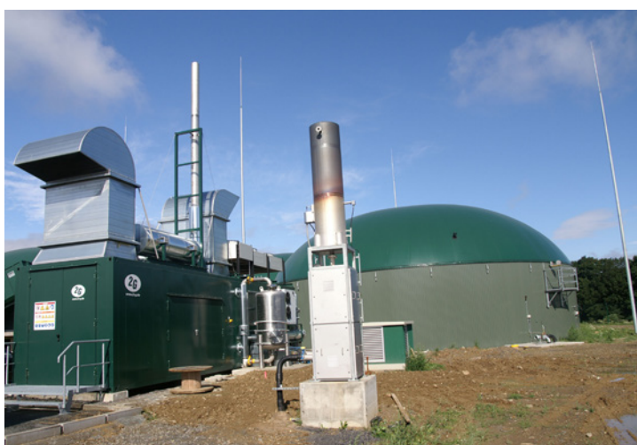
Figure 3.2 (a) Continuous stirred tank reactor (© Martin Dotzauer (DBFZ))
