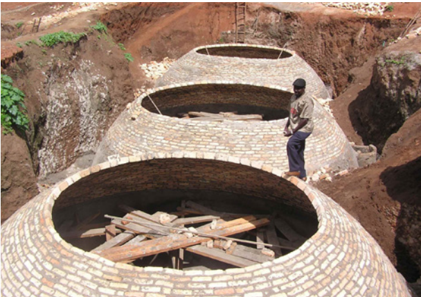
Figure 5.8 (a) Building underground domes Source: Ashden ( www.Ashden.org )
