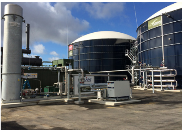
Figure 5.2 (a) Digesters and gas management Source: Biogas Renewables
