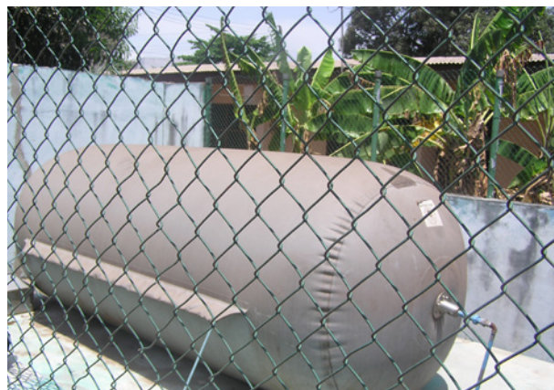
(b) Biogas stored in flexible bags
