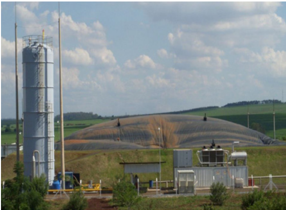
Figure 5.4 (a) Overview of the Ester biogas plant desulfurization tower (left), lagoon-based UASB reactor (left, behind), and CHP system (front) Source: Omnis Biotechnology
