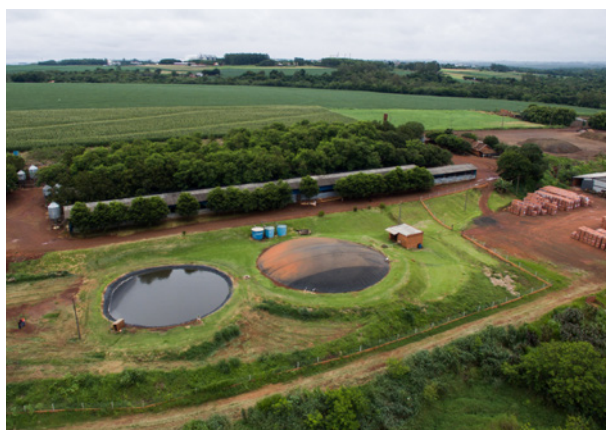
Figure 5.3 (a) Covered anaerobic lagoon Source: Cibiogas
