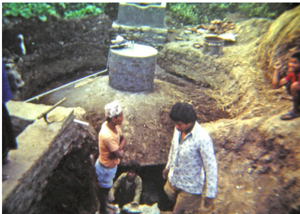
(b) Construction of fixed dome underground digester.
