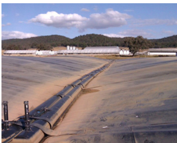
Figure 5.1 (a) HDPE covered anaerobic lagoon Source: Pork CRC Bioenergy Support Program
