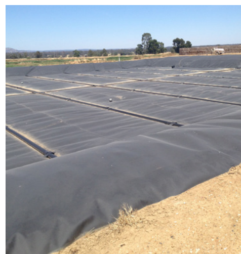
Figure 3.2 (b) Covered anaerobic lagoon (source: Pork CRC Bioenergy Support Program)
