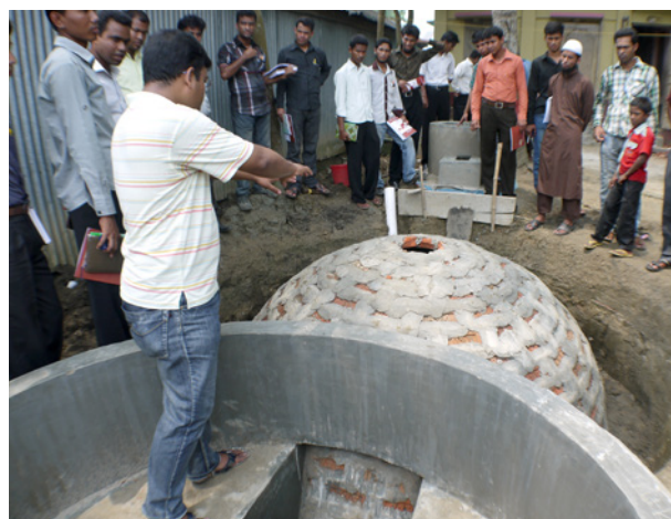
(b) construction of underground biogas plants
