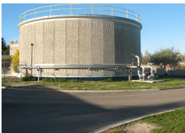
Figure 5.7 (a) Digester with mixing system for co-digestion of primary sludge, grease trap waste, and dairy factory DAF sludge.
