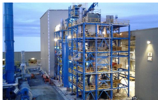
Figure 5: Ensyn Côte-Nord Biocrude Facility
