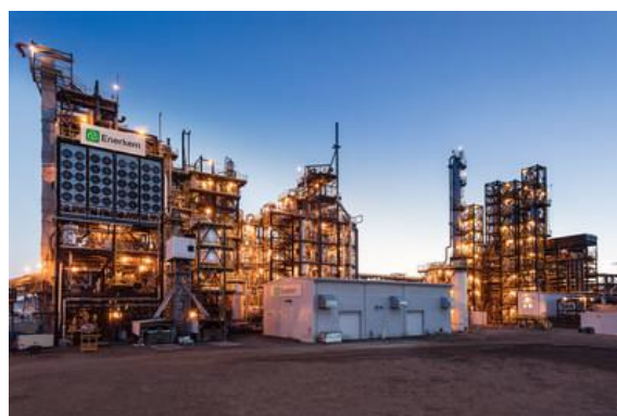
Figure 6: Enerkem Alberta Biofuels Facility
