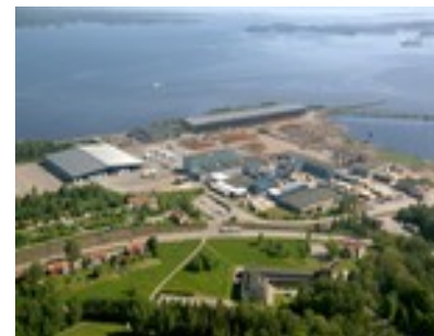
Pyrocell Setra, Gävle Sweden
