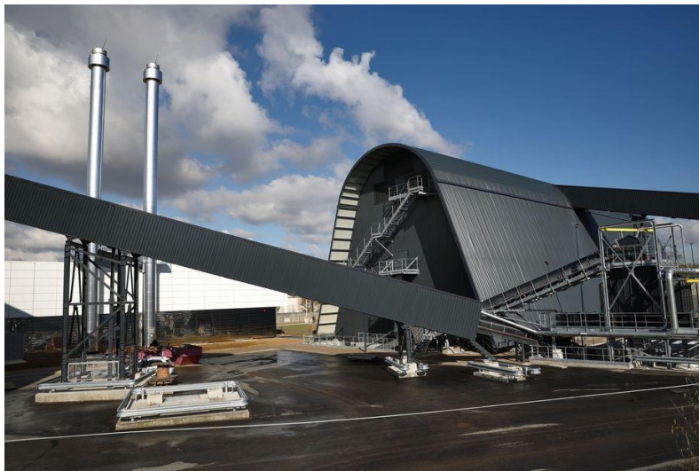
34 MW biomass heating facility in Lyon. https://www.usinenouvelle.com/
