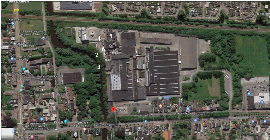
Figure 4. Google Earth image with the situation of the plant in its surroundings
