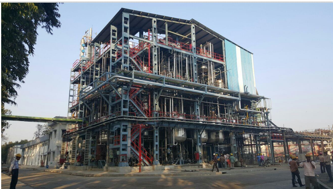
The 10 ton biomass/day Lignocellulosic ethanol plant at India Glycols Ltd., site at Kashipur, Uttarakhand, India built with the DBT-ICT 2G-Ethanol Technology
