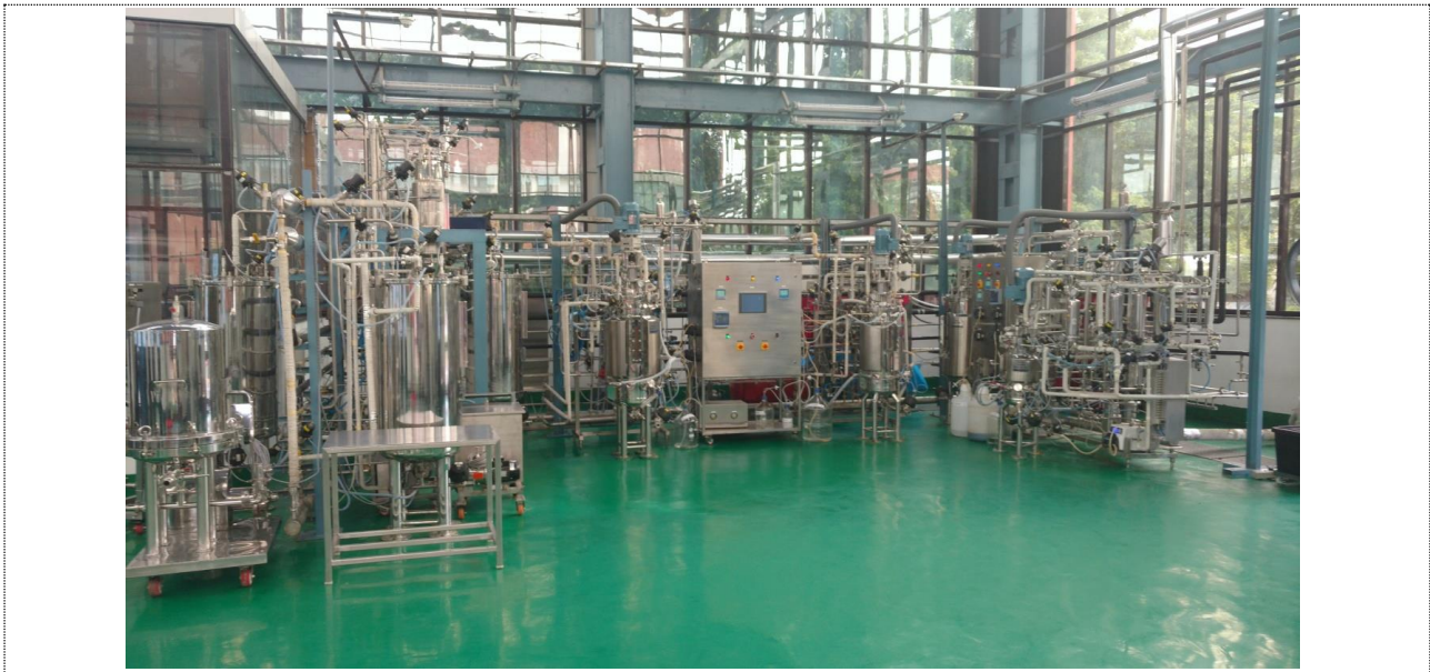
Carbon dioxide to high value lipids Pilot Facility, IndianOil R&D Centre, Faridabad, India
