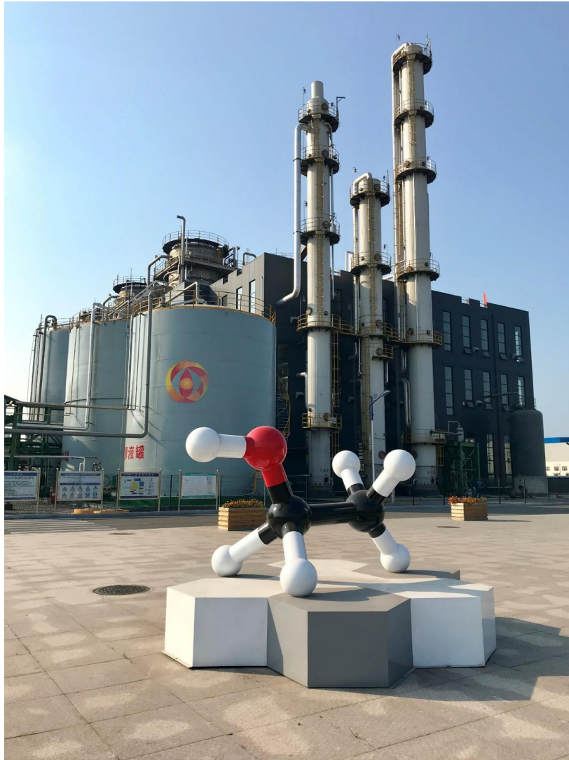
LanzaTech Commercial Facility with Shougang, China
