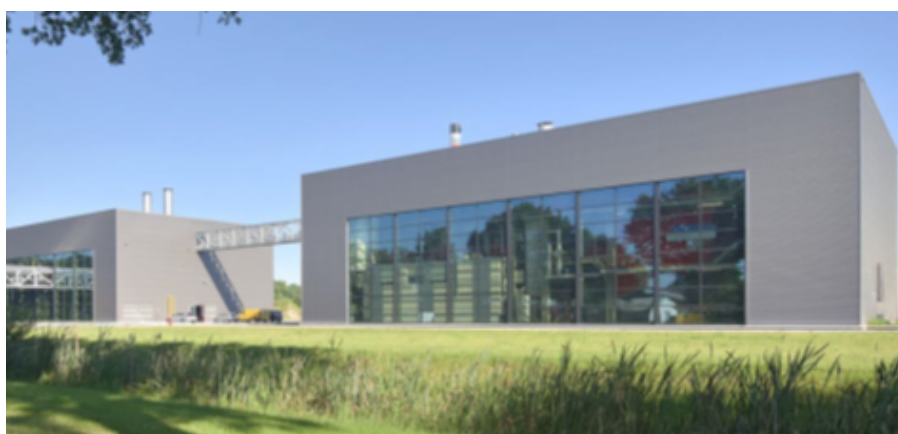
Figure 3: Process steam generation from wood chips and composting residues for potato processing in the Netherlands (source: Attero)
