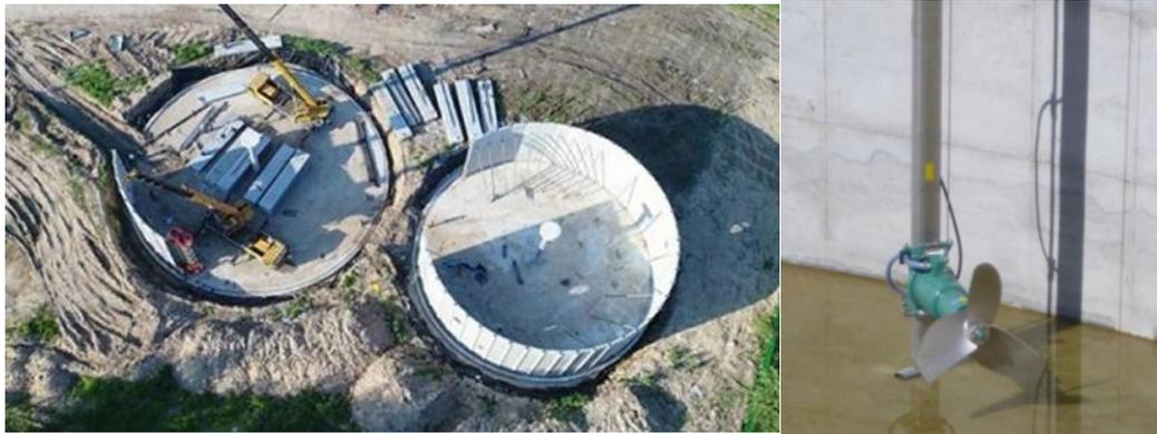
Figure 4: Erection of the fermenters (left), and submersible mixer (right)
