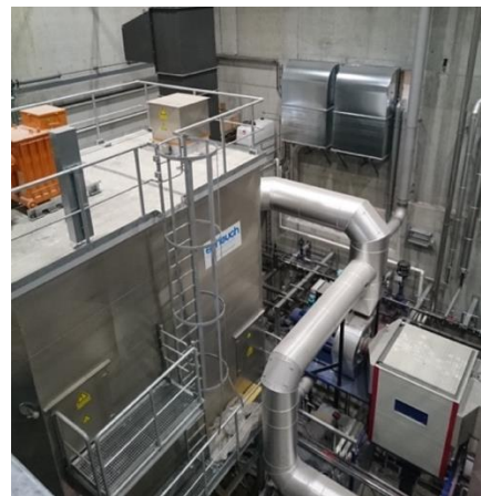
Figure 4. Boiler (KCO Kohlbach) with SNCR (ERC) (left) and electrostatic precipitator (Scheuch) (right).
