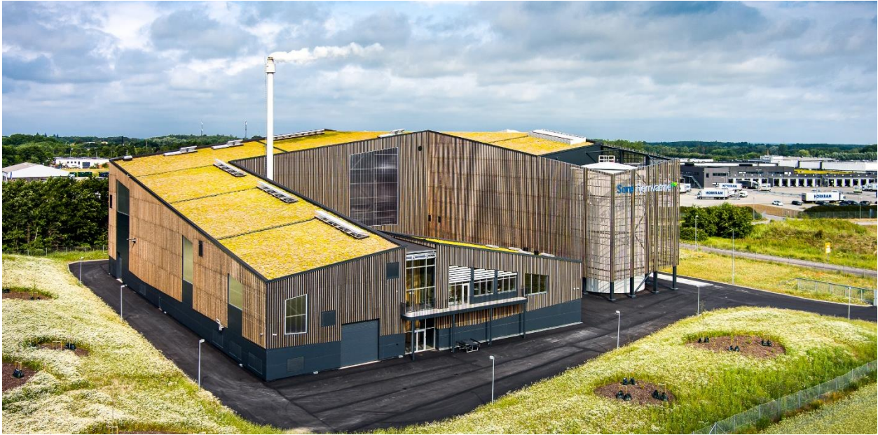
District heating plant in Sorø, Denmark (Photo: Steen Knarberg).
