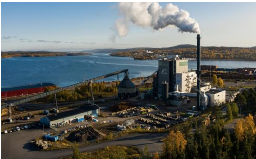
Liquid Wind's e-methanol production facility , Sweden (Figure: Övik Energi)
