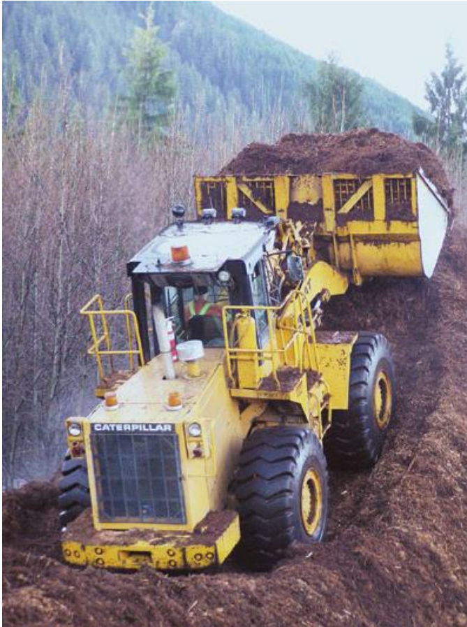
Figure 23 - Rubber tyred front end loader (RTFEL) piling hog fuel
