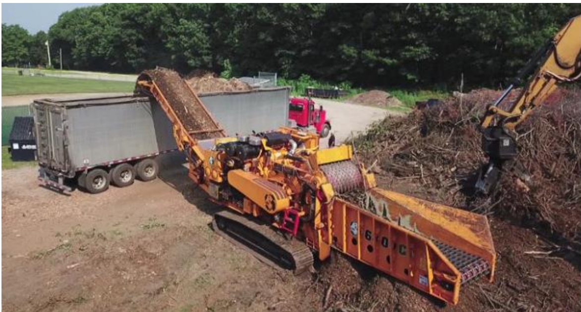
Figure 20 - mobile hogger (track mounted) loading direct to a truck
