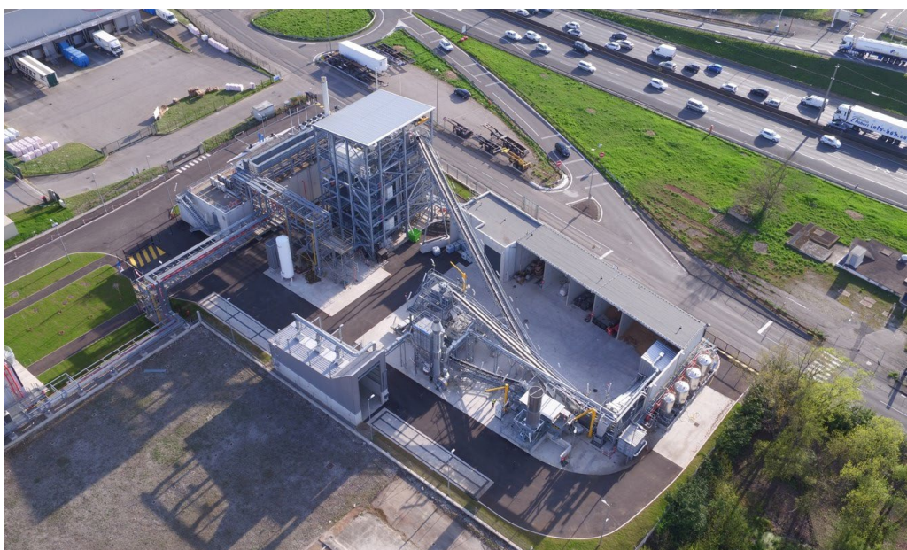
GAYA demonstration plant, south of Lyon © TBM-Technology Based Magic
