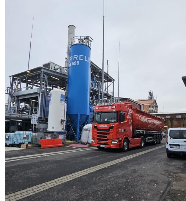
Suction Silo Truck docking at ARCUS-PDU Fine Dust Silo
