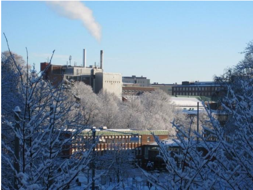
12 MW research boiler
