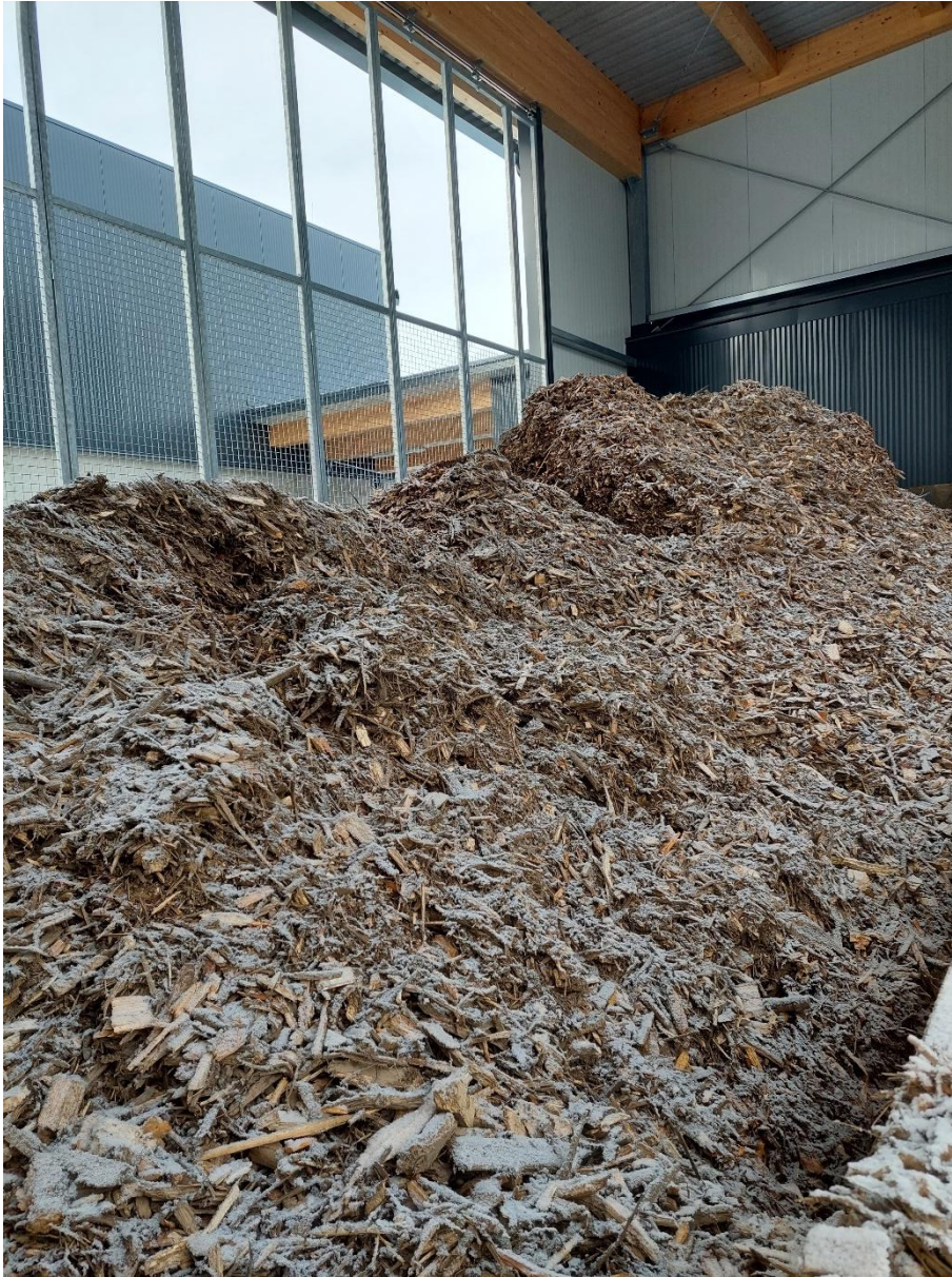
Figure 4: Fuel (forest residues) on moving floor storage (Source: BC Regionalwärme Group)
