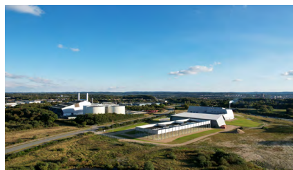
Silkeborg District Heating in Denmark has just recently commissioned a hybrid plant where an advanced biomass boiler system and a large air-to-water heat pump system benefit from each other to increase their efficiency/COP. (Photo: Martin Schubert, Arkikon).
